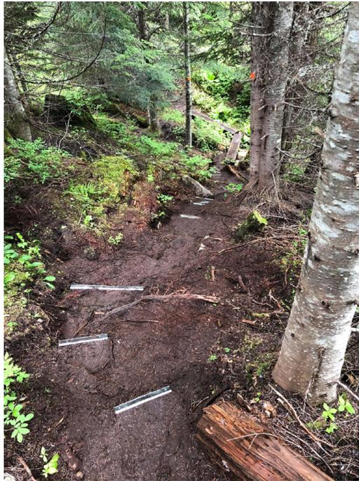
*We performed major upgrades and additions to the steepest sets of ramped steps in the connector trail at KM 1.2 These new steps use larger re-bar, longer beams of lumber, and are capped by fancy steel traction bars.*
