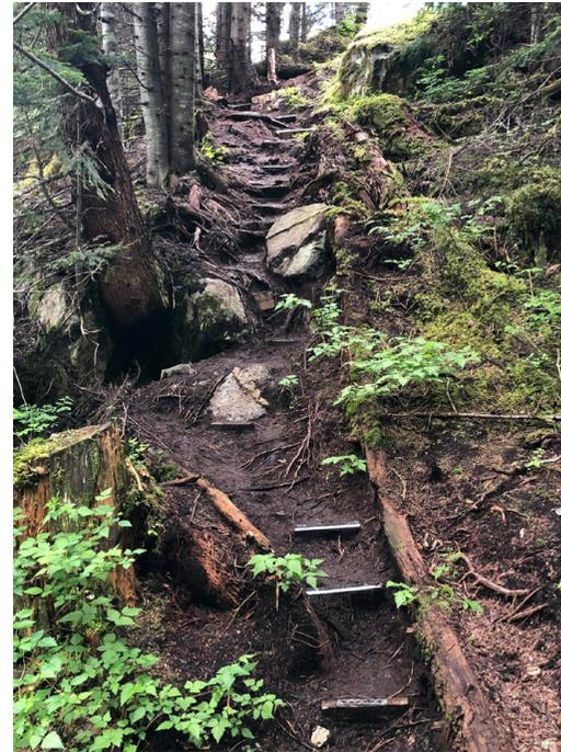
*Another steep section of steps in the connector trail. They are now more numerous, wider in some cases and capped with steel traction plates as well.*
